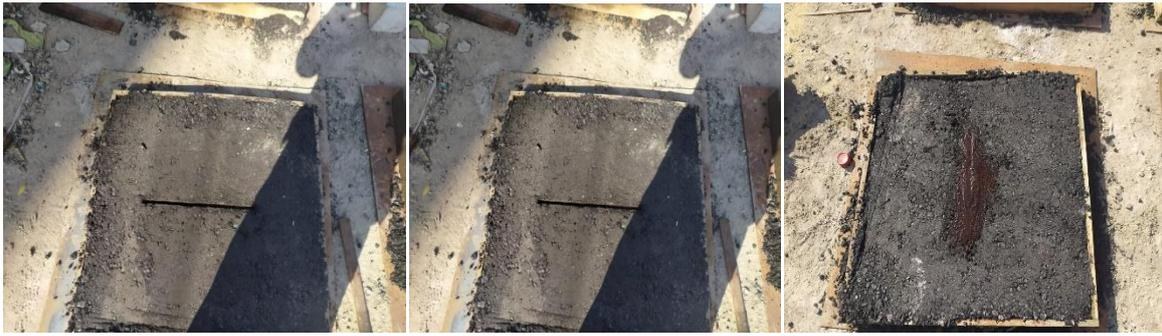
**Fig. 4. Steps of filling up of crack with cutback bitumen RC-70 with sand**
