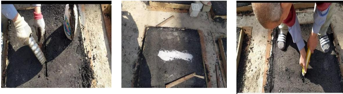
**Fig. 5. Steps of filling up of crack with Sikaflex®-1a**
